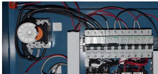
The fuse protection - breakers. (Illust. 16)
